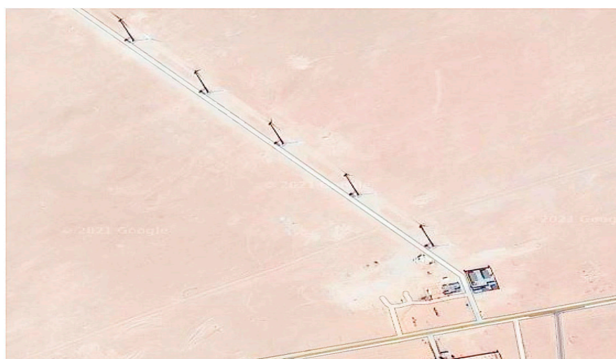
Figure 17. Typical configuration of twelve wind turbines ( 12 \times 0.85 MW) at Kaberten wind farm.
