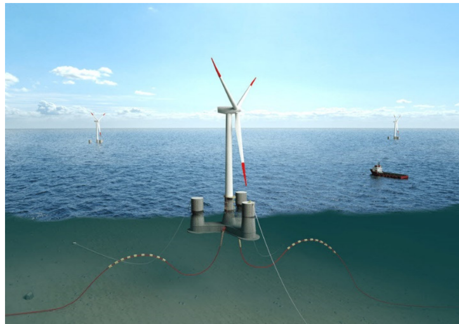
Figure 1. LIFES50+ OO-Star Wind Floater Semi 10 MW.
