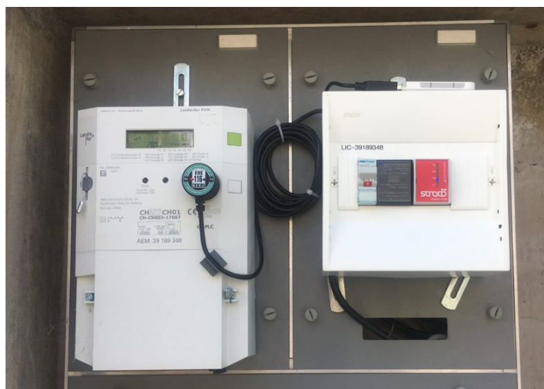
Figure 2. Strato Pi CM (right), USB 4G connection dongle (on the case of the Strato Pi CM) and smart meter (left) with optical reading probe, installed at a point of delivery.
