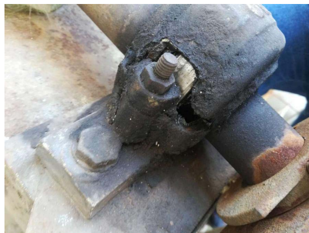
Figure 3. The diagram of the base cracking of the exhaust fan blade actuator.
