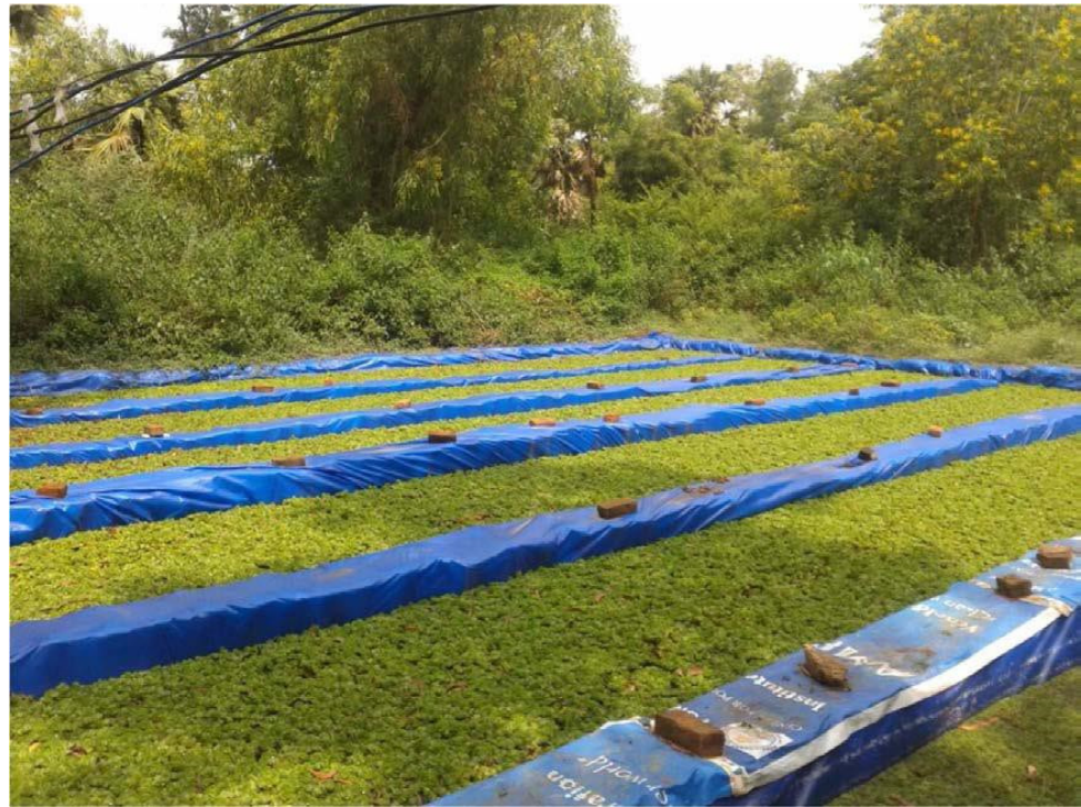
Figure 2. Another SHEFROL plant treating sewage continuously. It is planted with Salvinia molesta .
