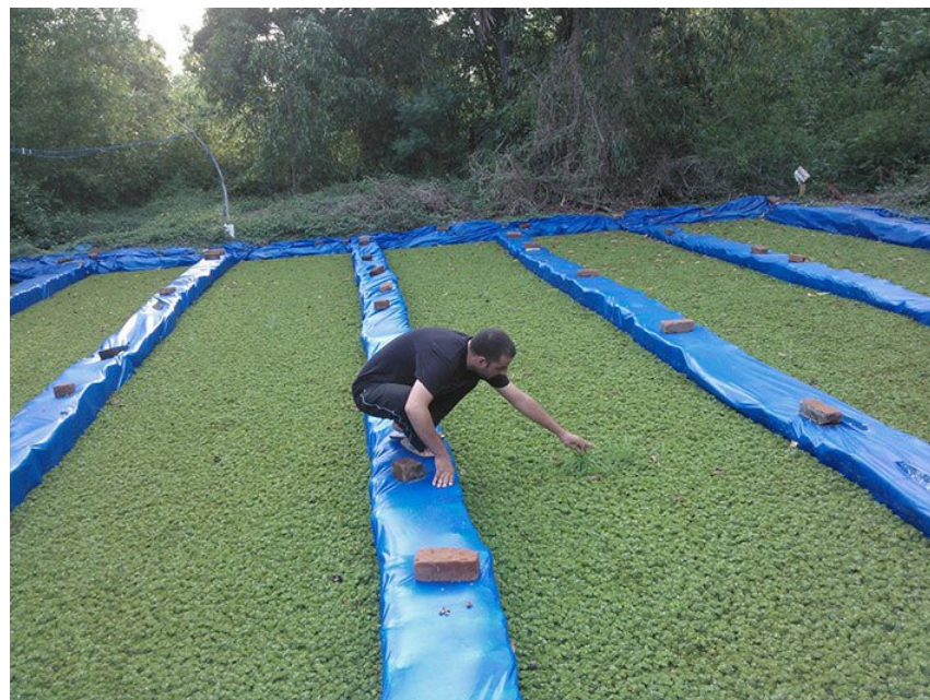
Figure 1. A typical SHEFROL plant treating sewage with duckweed as the main bioagent.
