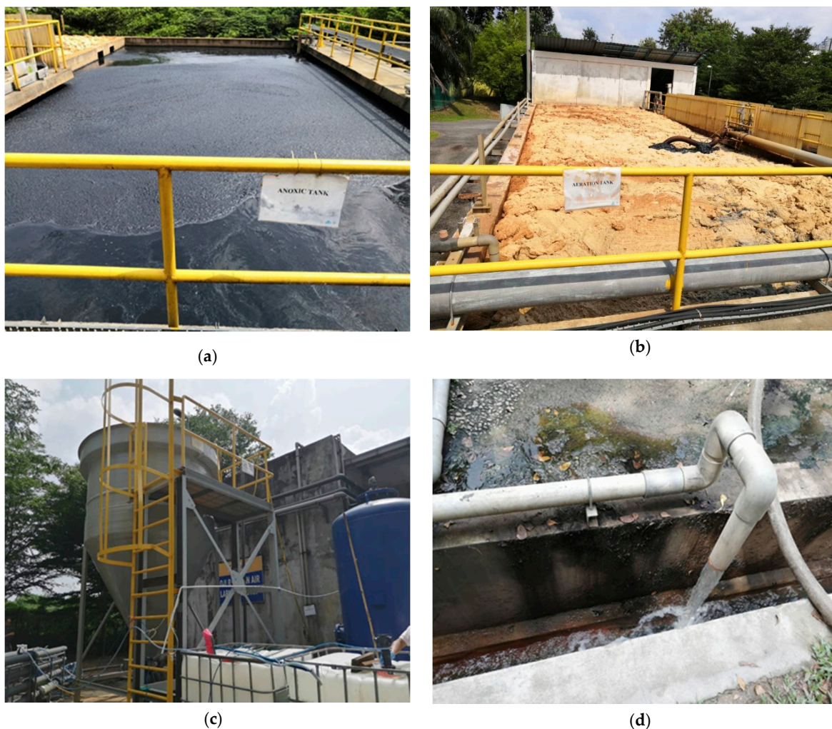
Figure 4. Sampling points. (a) Anoxic tank, (b) aeration tank, (c) secondary clarifier tank, (d) final discharge point.
