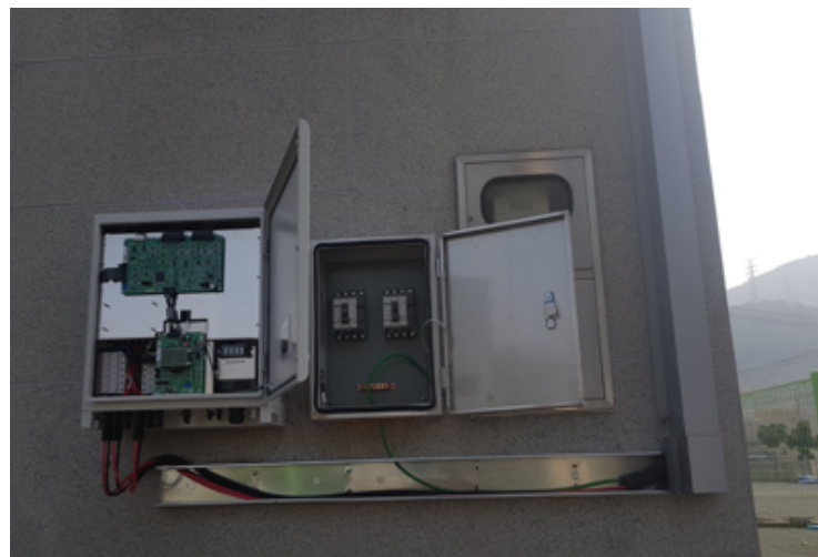
(b) Inverter and junction box.
