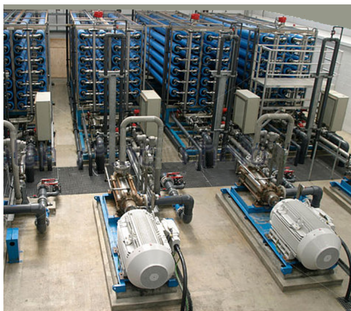
Figure 5. RO racks of an industrial seawater RO desalination plant.
