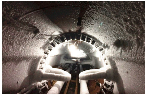
Figure 4. Interior of Hollow Pipe showing Profiled Freezing-Tube.
