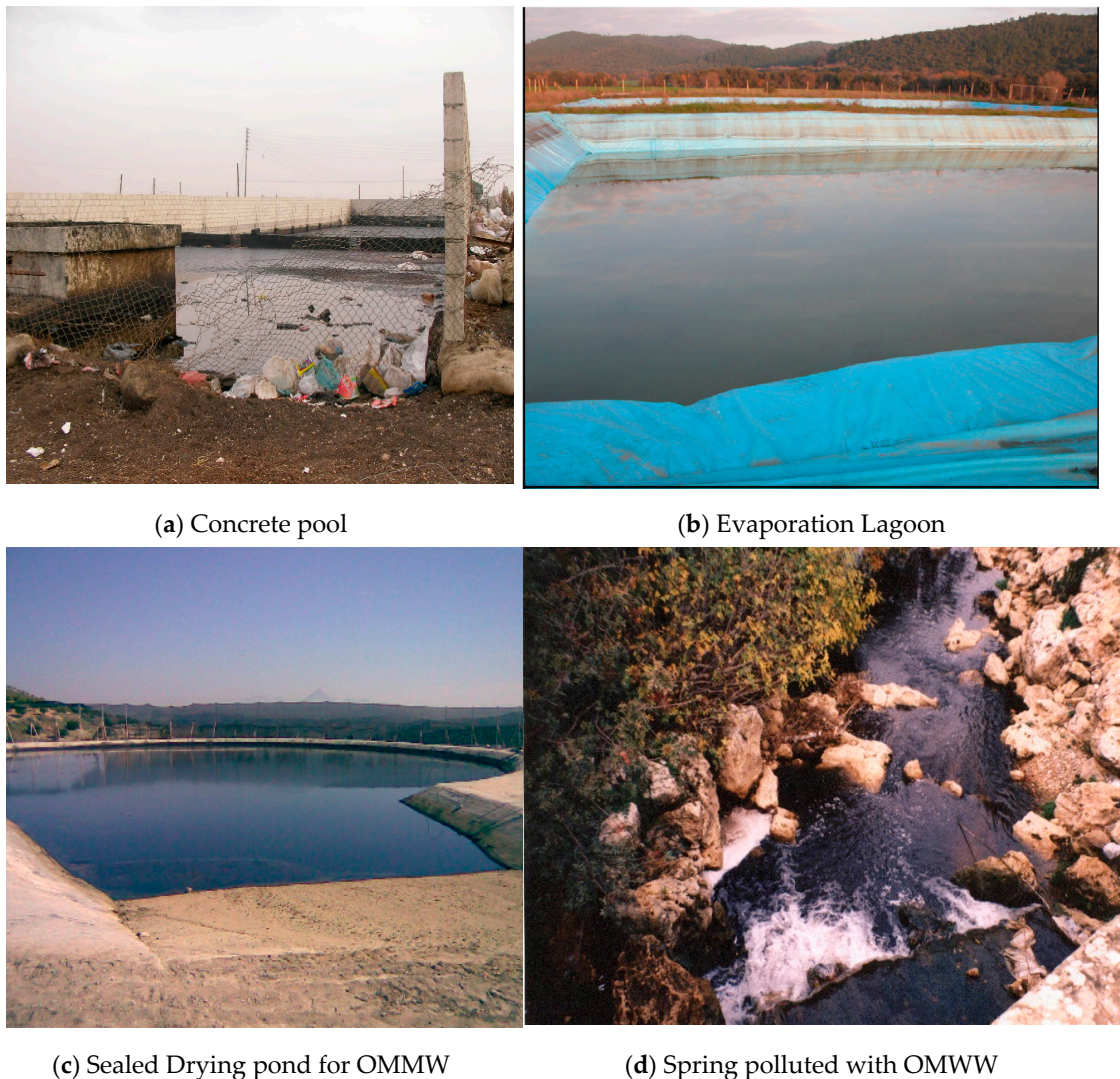
Figure 2. Wastewater storage and handling at different locations of olive mills in Irbid area.
