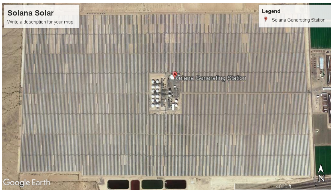
Figure 6. Google Earth view of Solana solar energy project. Map data ©2020 Google.
