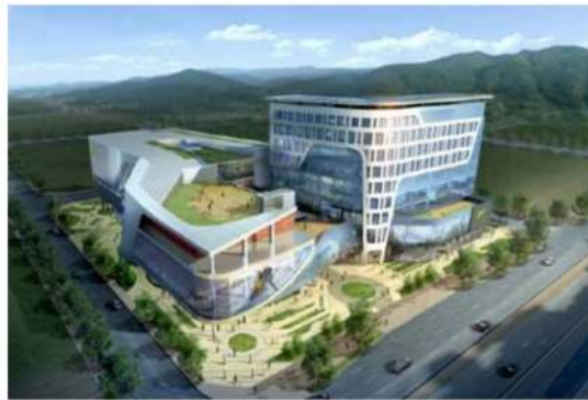
Figure 1. Exterior of the building.
