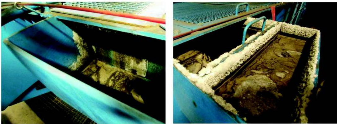
Figure 6. Tribocorrosion traces on the walls of deslagger water trap occurred during operation with high temperature water in the tub.
