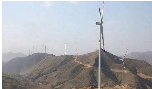
Figure 5. 100 KW medium-size wind turbines from a wind farm in Henan.
