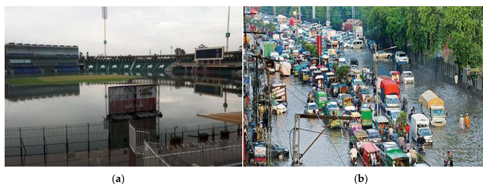
Figure 2. (a) Ponding condition inside Gaddafi Stadium; (b) a traffic mess on Circular road after rainfall (DAWN news)
