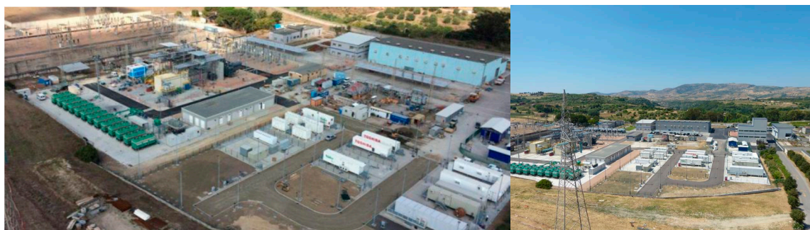
Figure 3. Two views from above the Codrongianos substation.
