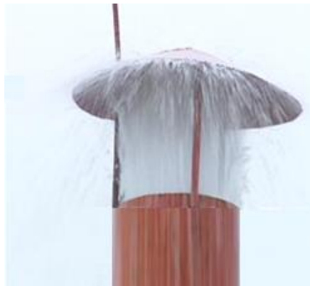
Figure 12. Gas jet at the ground 2# drainage borehole.
