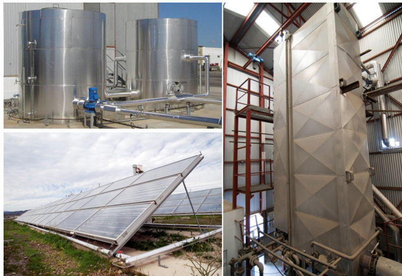
Figure 2. Solar desalination facility at PSA-CIEMAT. From left to right and from top to bottom: cold and hot tanks, MED unit and solar field.
