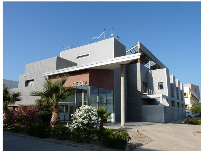
Figure 6. The CIESOL building.
