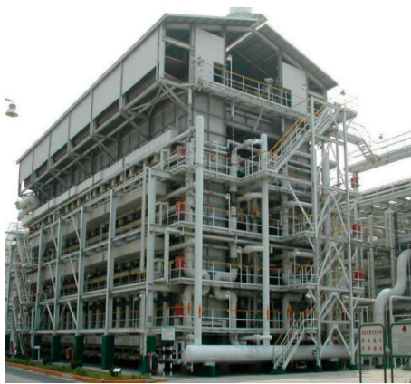
(a) a typical steam methane reformer
