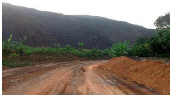
Figure 2. Disposal site of Khanh Hoa coal mine has reached 250 m in height and significantly altered provincial geomorphology.
