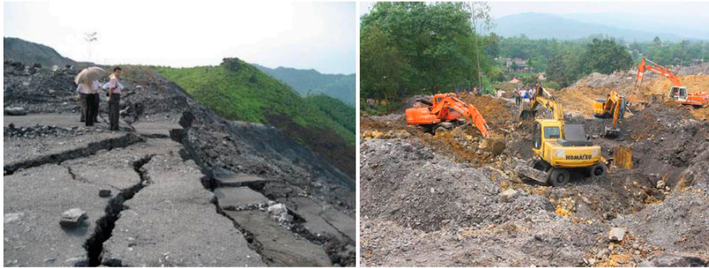
Figure 4. Heavy rains in April 2012 caused landslide at slag heap of Phan Me coal mine, killing 5 people and burying 10 houses.
