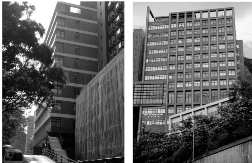
Figure 2. The CYC building: north façades (left) and south façades (right) (Photo by authors).
