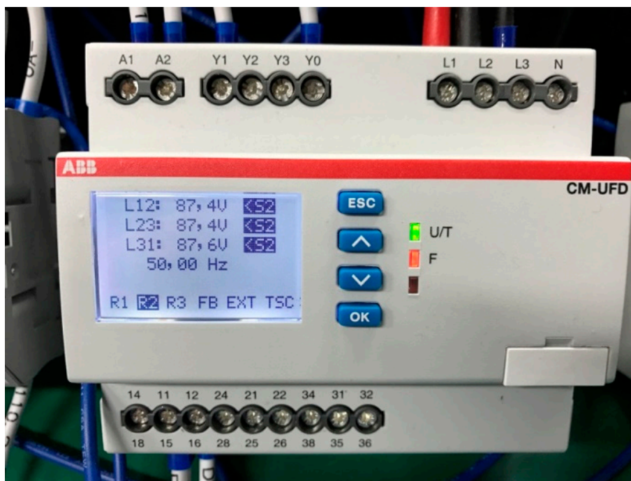
Figure 28. Under voltage relay operation.
