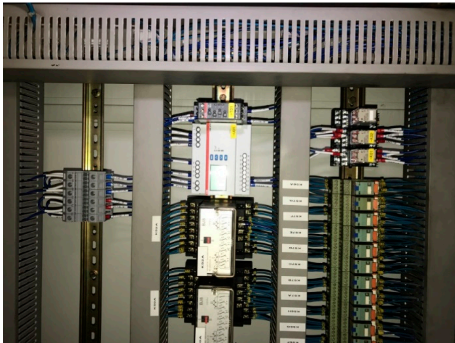
Figure 33. The panel after installing the relay.
