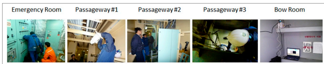
Figure 16. Ship power line communication installation process.
