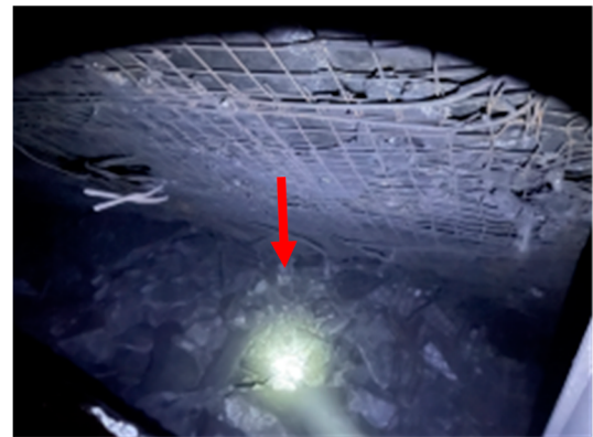
(b) Roof cutting.
