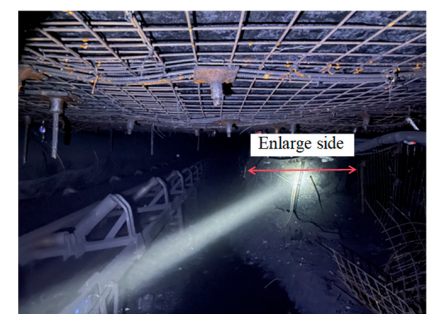
(c) Enlarged entry side for repairs
