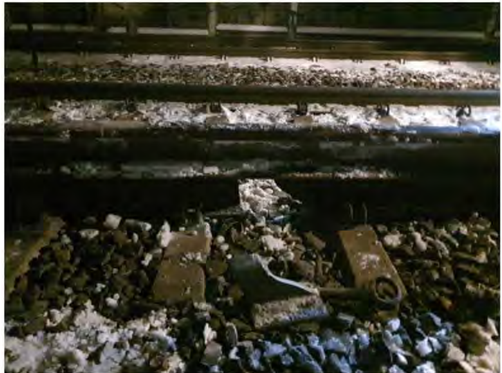
Figure 1. Rail cracking due to low temperatures (source: photo made by Jacek Makowski).
