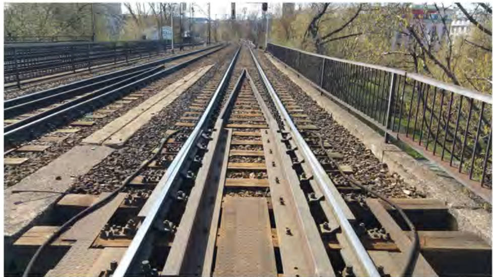
Figure 5. Breathing section of track No. 2 at km 2.100 (source: photo made by Jacek Makowski).
