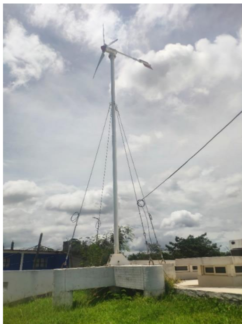
Figure 1. RTO-1kW Wind Turbine, installed in the Ejidal Bioclimatic Community Center of La Venta, Oaxaca, Mexico.
