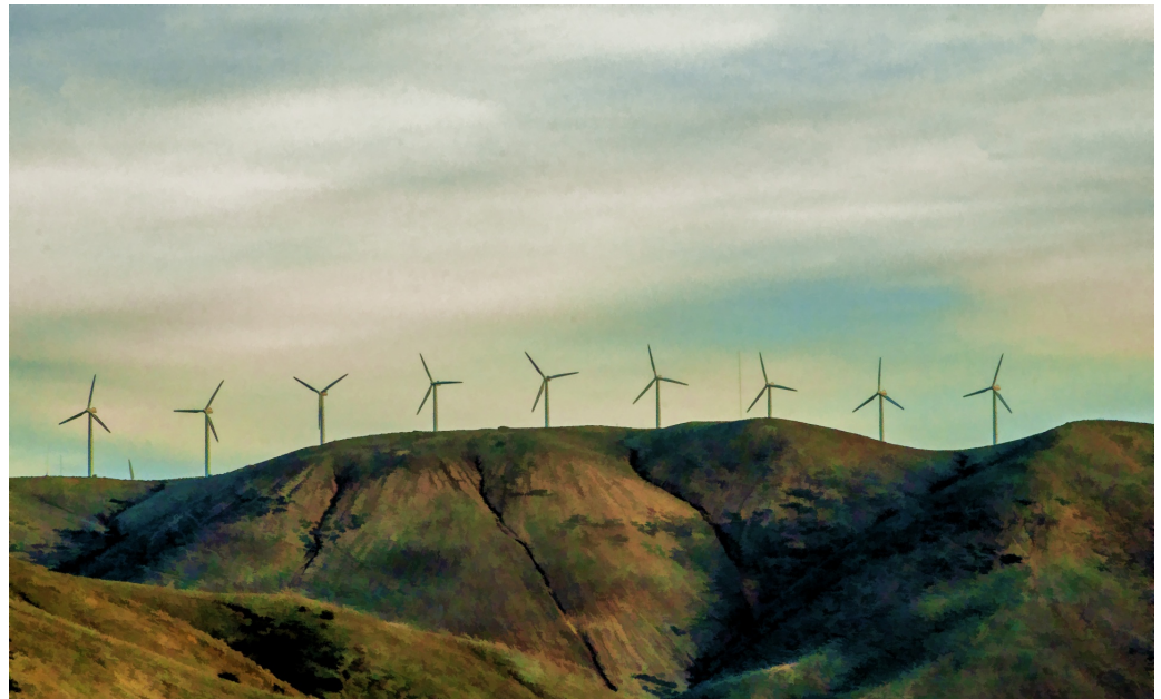
Figure 3. View on one of the wind farms. Source [34].
